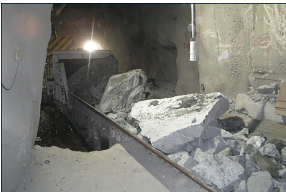
Large feed material on the chain conveyor in front of crusher inlet (copper ore, underground)
